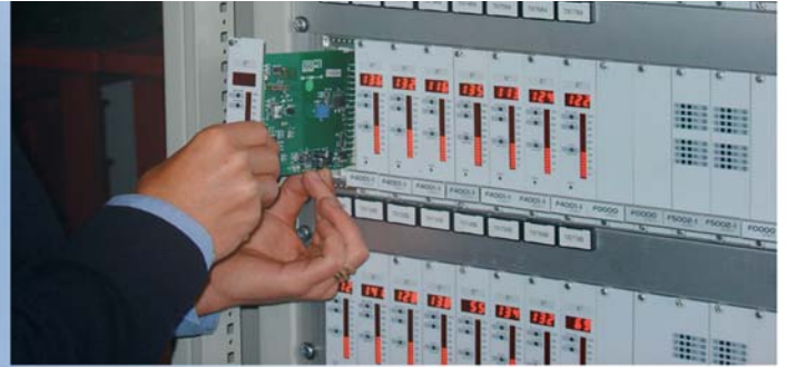
Hot swap of cards, with consequent no need for panel shutoff
