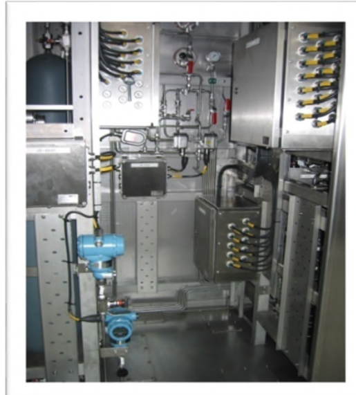
Junction Boxes in Common Section
